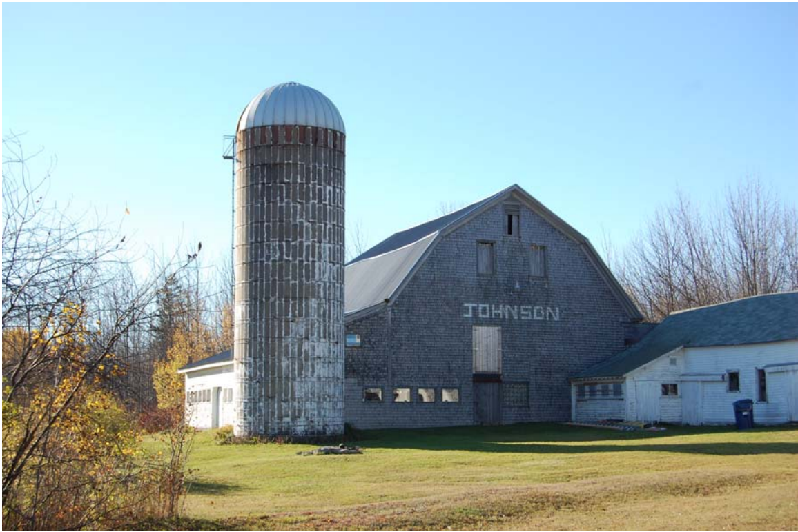
Photo 7: 166 North Road barn and silo.
