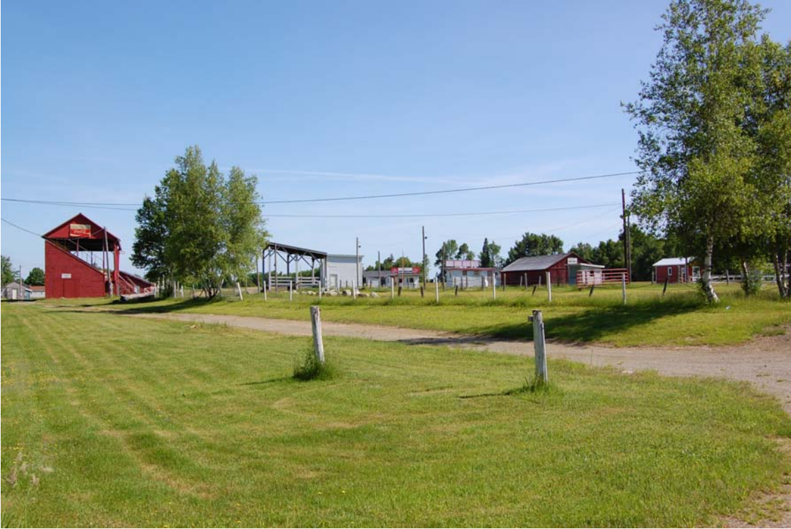
Photo 4: Springfield Fairground buildings.
